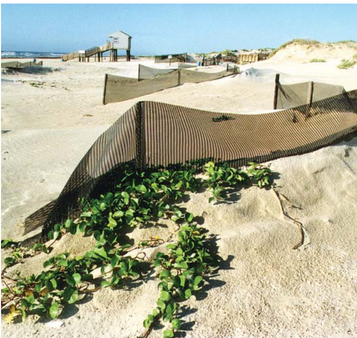
Figure 17. Sand fencing used to trap sand.
