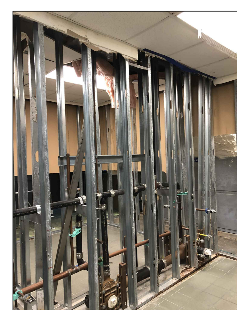
PHOTOS ARE EXISTING CONDITIONS FOR REFERENCE ONLY
