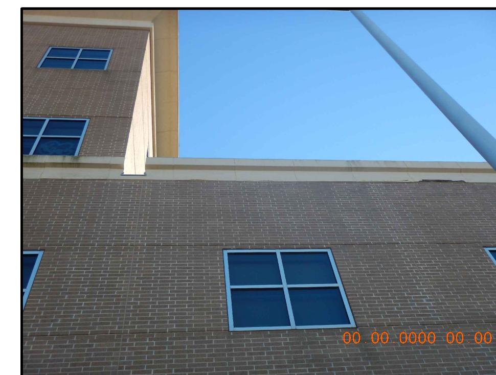
EIFS TO BE REPLACED AT THE MID-HEIGHT TRIM & PARAPET TRIM W/GFRF. RE: DETAILS 2 & 3
