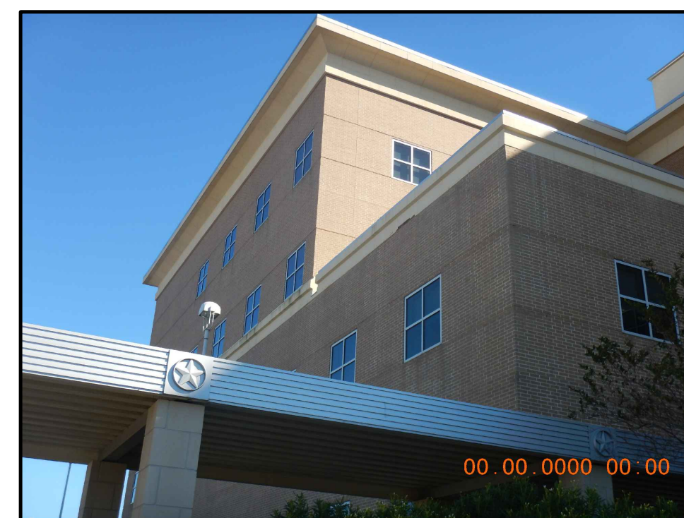
EIFS TO BE REPLACED AT THE MID-HEIGHT TRIM & PARAPET TRIM W/GFRF. RE: DETAILS 2 & 3
