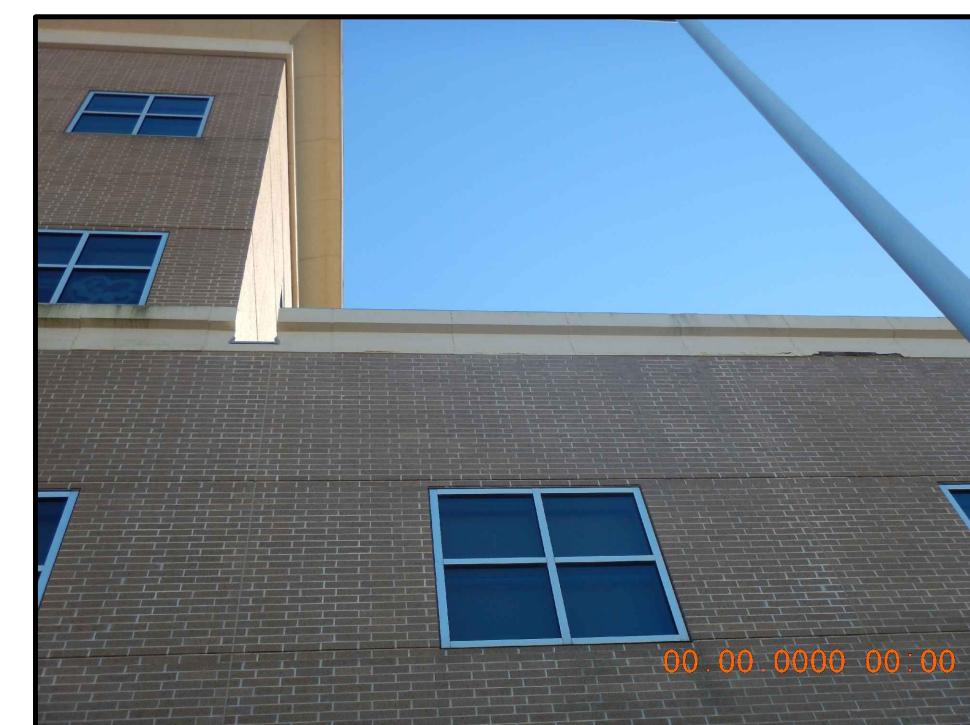
EIFS TO BE REPLACED AT THE MID-HEIGHT TRIM & PARAPET TRIM W/GFRc. RE: DETAILS 2 & 3
