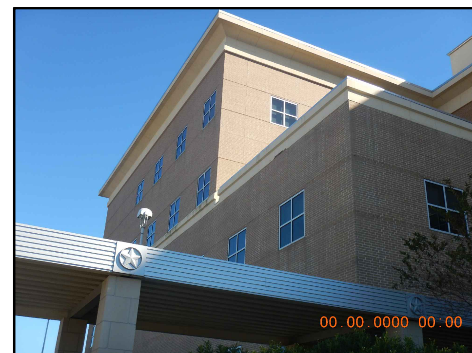
EIFS TO BE REPLACED AT THE MID-HEIGHT TRIM & PARAPET TRIM W/GFRc. RE: DETAILS 2 & 3
