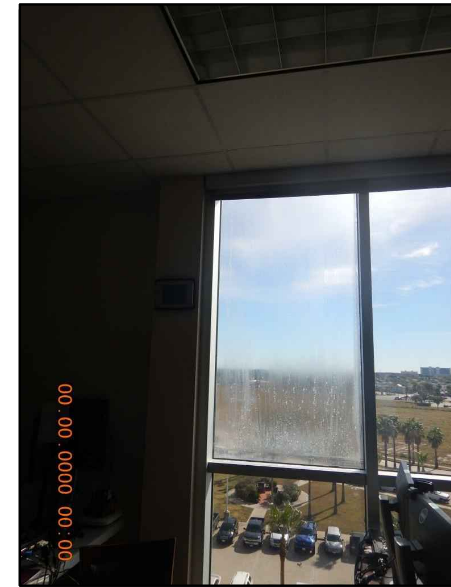
PHOTO A - WINDOW ON 3RD FLOOR
