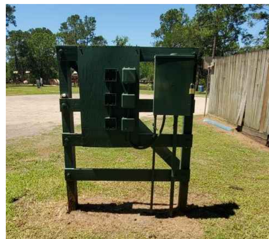
3 SITE 6 EXISTING REFERENCE PHOTO NTS
