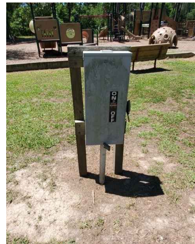
3 SITE 2 EXISTING REFERENCE PHOTO NTS
