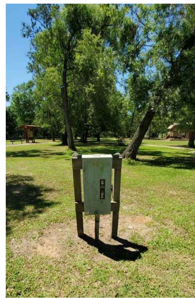
3 SITE 4 EXISTING REFERENCE PHOTO NTS
