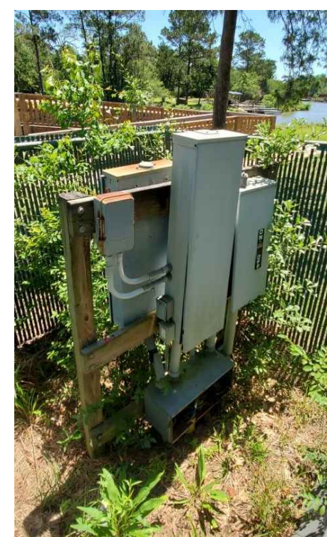
3 SITE 1 EXISTING REFERENCE PHOTO NTS
