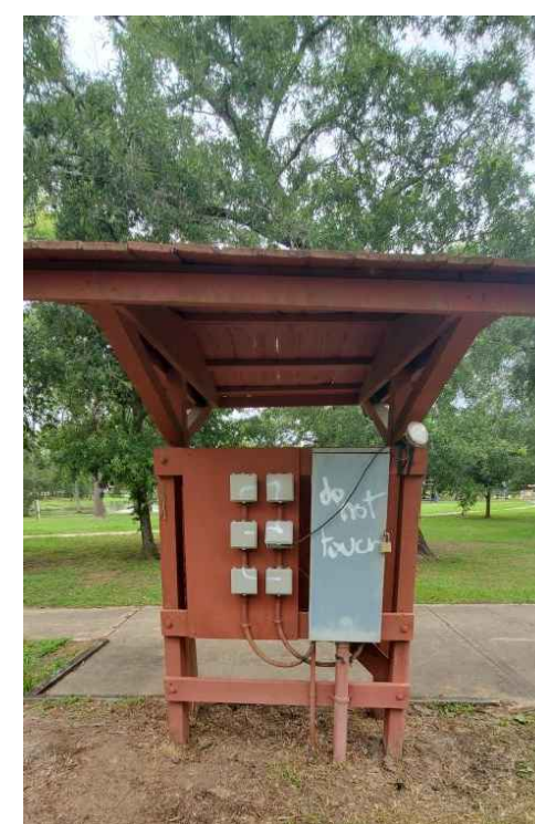
3 SITE 3 EXISTING REFERENCE PHOTO NTS
