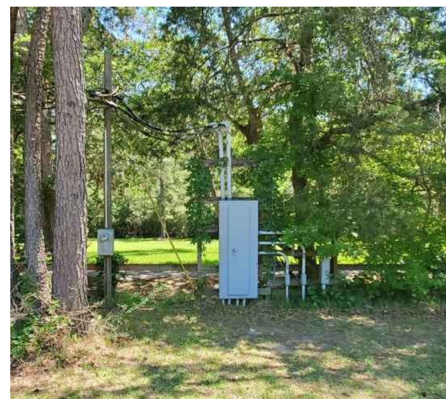
3 SITE 7 EXISTING REFERENCE PHOTO NTS
