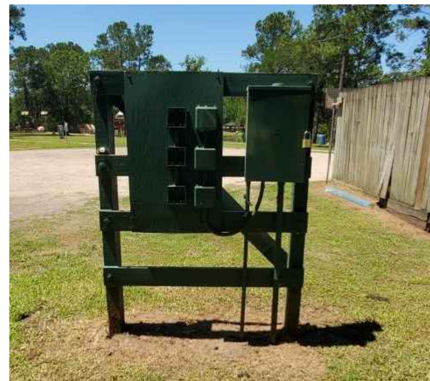
3 SITE 6 EXISTING REFERENCE PHOTO NTS
