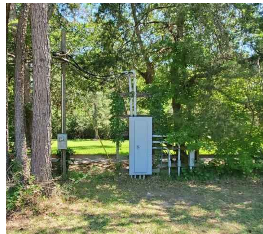
3 SITE 7 EXISTING REFERENCE PHOTO NTS
