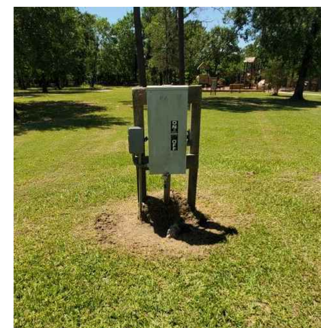
3 SITE 5 EXISTING REFERENCE PHOTO NTS
