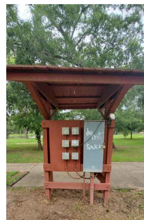
3 SITE 3 EXISTING REFERENCE PHOTO NTS
