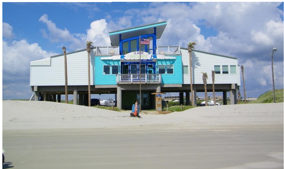
New Restroom / Concession Building
