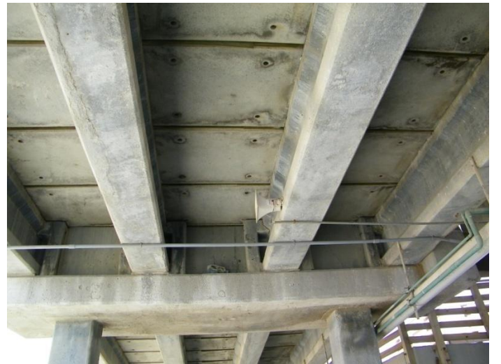
Horace Caldwell Pier and IB McGee Beach Park
