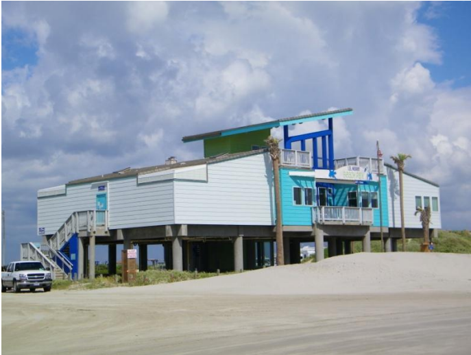
New Restroom / Concession Building
