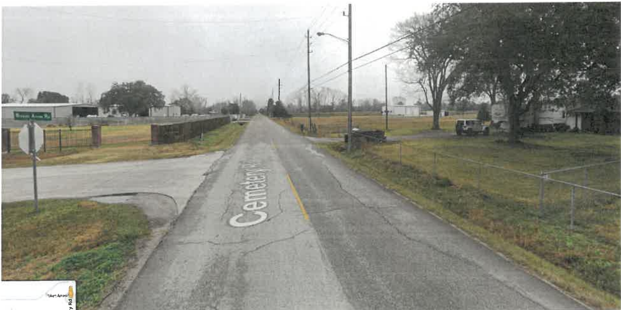
Cemetery Rd - at Broken Arrow
