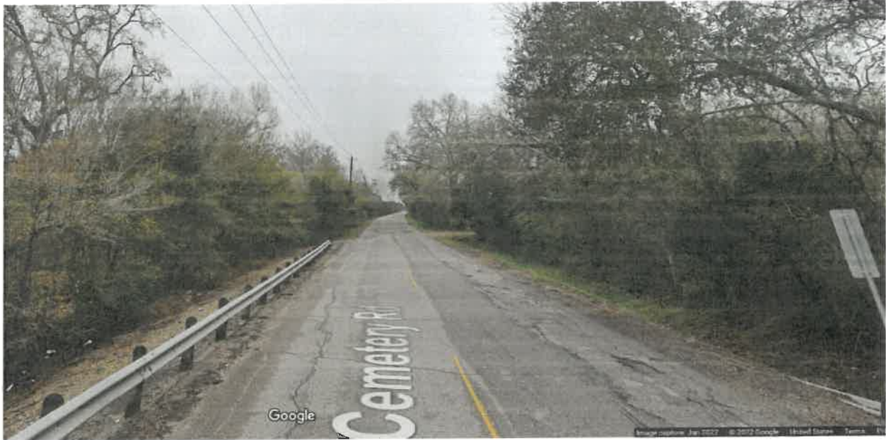
Cemetery Rd - North of Dickinson Bayou Bridge
