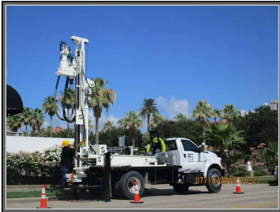
P-3 (A Picture of Drilling Operation along 23 rd Street)
