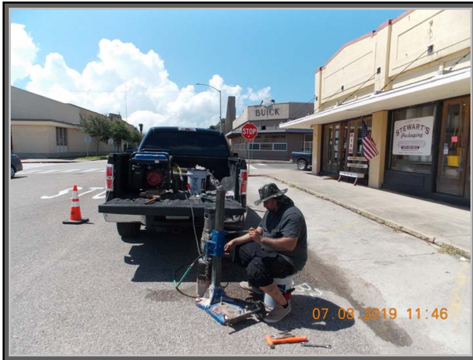
P-1 (A Picture of Coring Operation along 23 rd Street)
