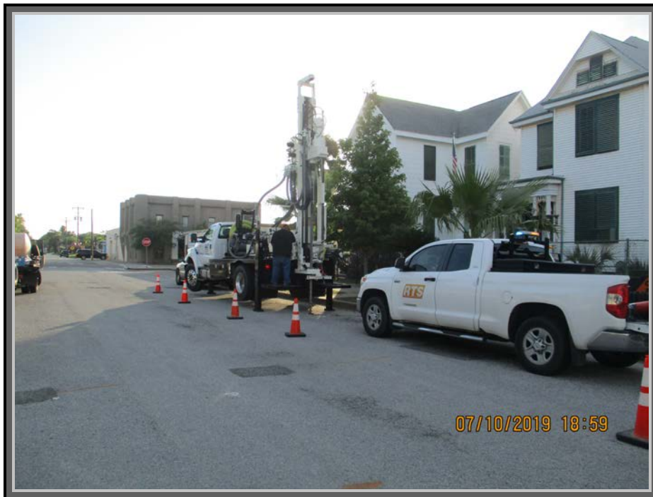
P-4 (A Picture of Drilling Operation along Avenue N)
