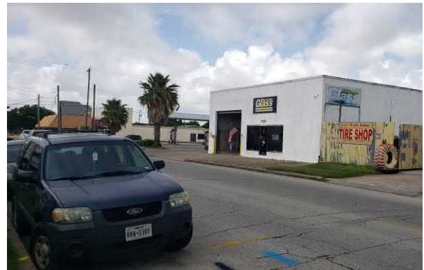
Photo 4 View of Binswanger Glass and a Tire shop (former auto repair), east of 53 rd Street
