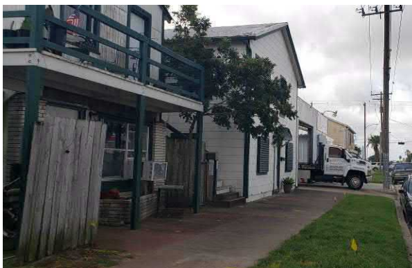
Photo 5 View of Gulfside Overhead Door (former auto repair) east of 53 rd Street
