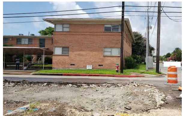
Photo 10 View of an apartment complex at the SW corner of Avenue S and 45 th Street
