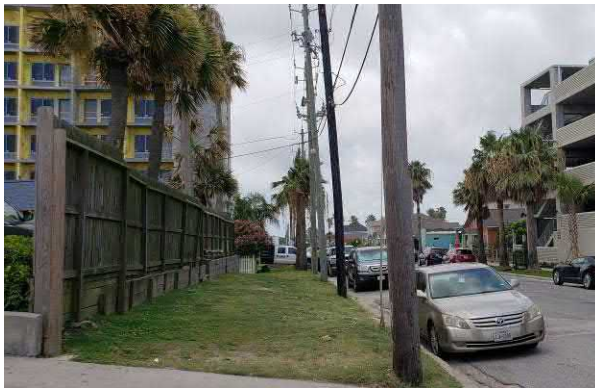
Photo 21 View of a parking garage located along Avenue S, west of 32 nd Street
